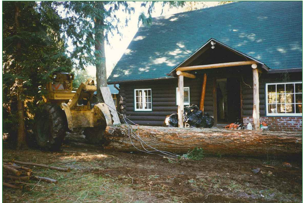
Heavy equipment was brought in to begin the restoration process
