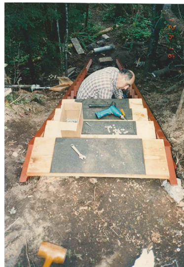
Terry building the steps down to the river.
