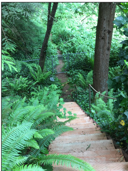
The finished steps down to the Sandy River.
